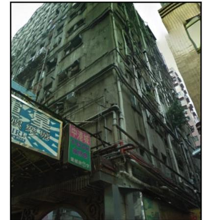
**Figure 4.12** Piping should not be clear to view
