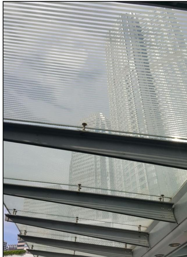
**Figure 3.30** Fritted glass and supporting structure detail
