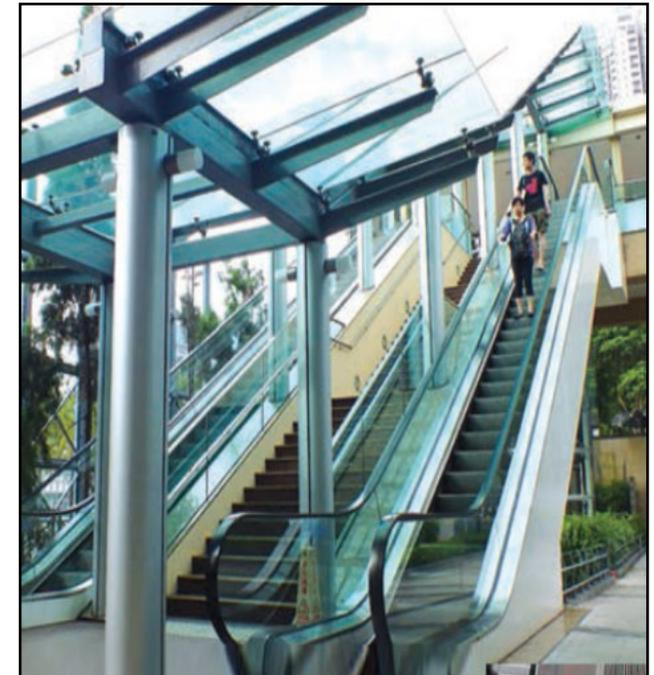
**Figure 3.39** In conditions where escalators located in external spaces, fritted glass canopies should be employed to provide all weather protection and ensure good illumination.
