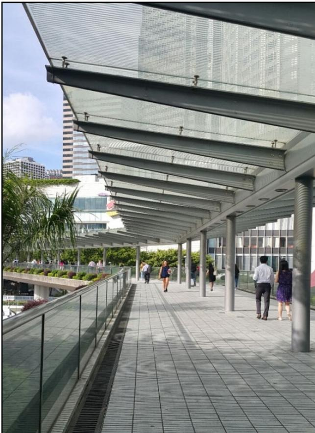
**Figure 3.29** Fritted glass canopy and balustrade combined to create a sense of “lightness” and provide visual porosity
