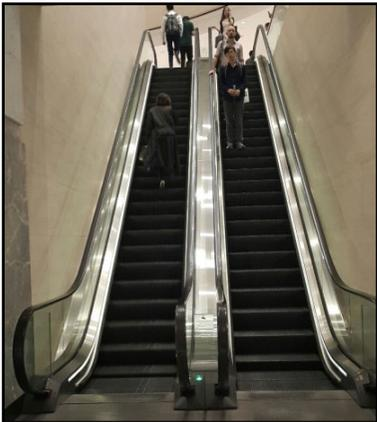
**Figure 3.32** Acceptable standard escalators with glazed edges
