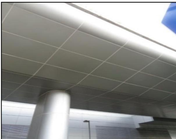
Figure 3.22 Underbelly of the recommended elevated connection should be clad in aluminium to match the underbelly cladding of the landscaped deck
